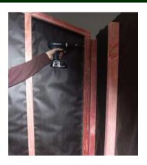
Step 6: Silicone edge of weatherboards on standing panel and nail on cedar beads with 5 x bead nails. (Refer to wall plan for correct beads). Make sure bead is properly sealed to avoid leaks.
