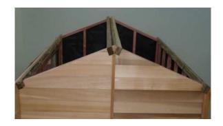
Step 14: Using 1 x 75mm tek screw, screw bottom purlin to top plate centrally in shed.
