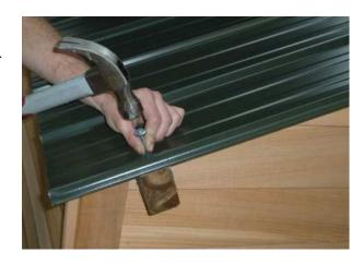
Step 17: Lay out remaining full roof sheets. Rivet these sheets together, 2 rivets per join, to make 1 large roof panel as shown in photo. Tack remaining top corner and bottom corner ensuring edge of sheet is flush with end of purlins and height is correct.
