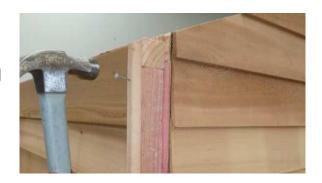
Step 12: Silicone and nail corner clashings on all corners as shown using 5 x bead nails per clashing.
